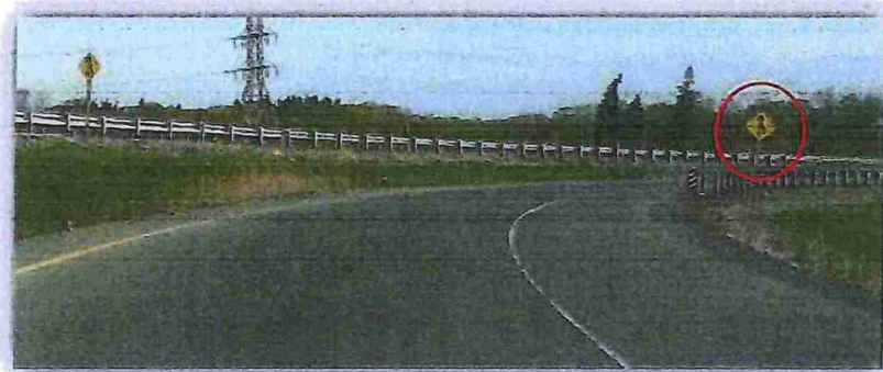
Figure 25 – Inappropriate Merge Warning Sign (View North from On-Ramp)
