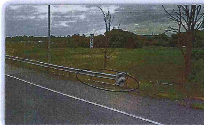
Figure 21 – Culvert and Ditch within Deflection Area of Approach Eccentric Loader End Treatment (View North from Beginning of Off-Ramp)
