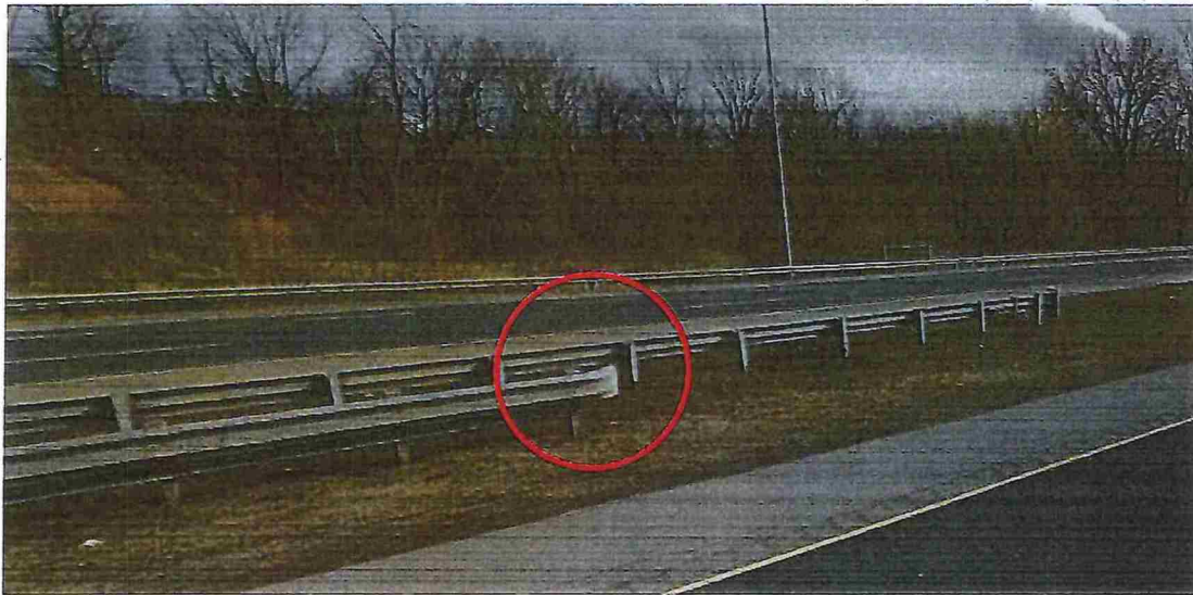
Figure 18: RHVP typical guide rail leaving end treatment
