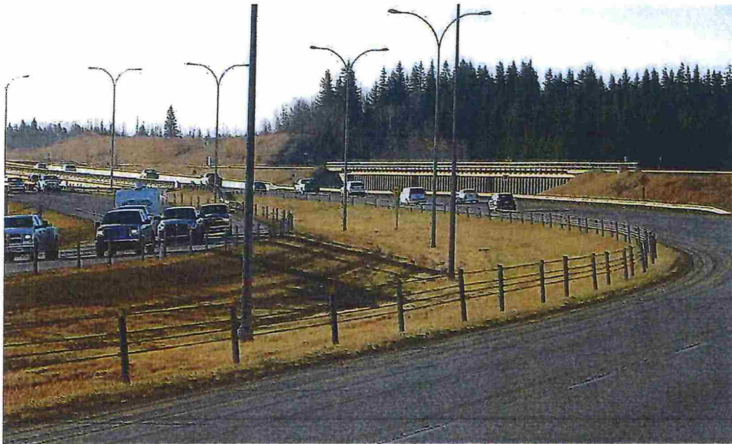
Figure 31: Example of high tension cable barrier
