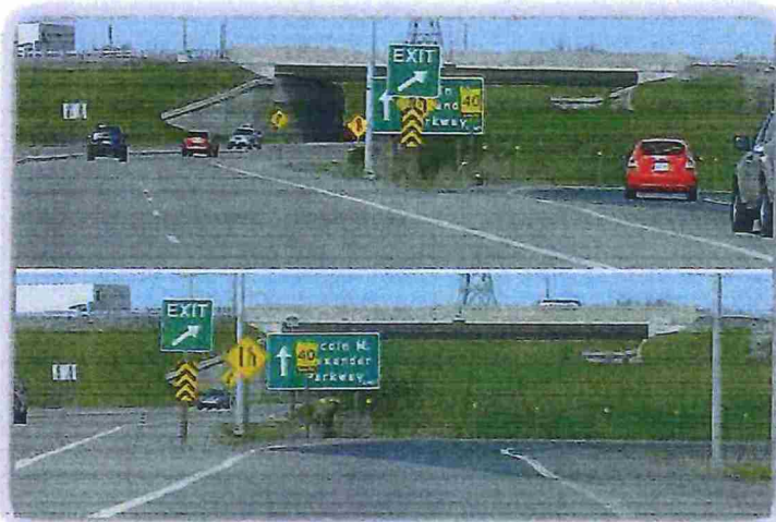
Figure 23 - Closely-Spaced and Eclipsing Signage (View West from Beginning of On-Ramps)
