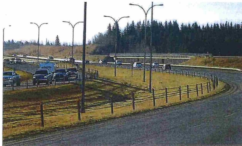
Figure 2 : An Example High Tension Cable Barrier
