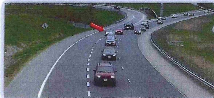
Figure 18 - Potentially Restricted Sightlines for Merging Traffic
