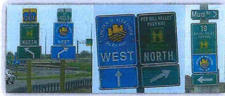
Figure 10 - Trailblazer Information Sign Displays (Various Locations Leading to RHVP/Link On-Ramps)
