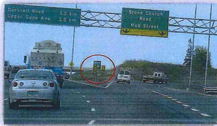
Figure 14 - Freeway Exit sign Partially Eclipsed by the Object Marker Warning Sign (View South from the Mainline)
