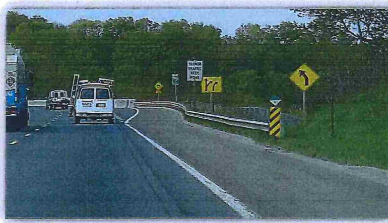
Figure 12 - Closely-Spaced Signage Upstream of the Stone Church Road and Mud Street Off-Ramp (View South from the Mainline)
