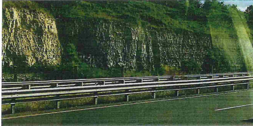
Figure 1: An Example Standard Steel Beam Guide Rail with Channel System
