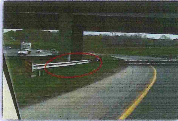
Figure 19 - Uneven Terrain Immediately In Front of the Steel Beam Guide Rail System (View North from the Mainline)
