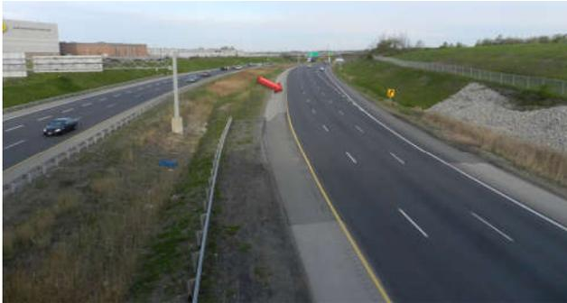
**Figure 15 - View of Discontinuity in Horizontal Curve on the Mainline (View West from Pritchard Road Overpass)**
