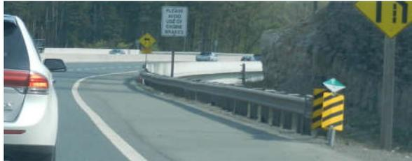
Figure 31 - Object Marker Damaged and Not Vertically Plumb (View North from the Mainline)
