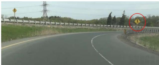
Figure 30 – Inappropriate Merge Warning Sign (View North from On-Ramp)
