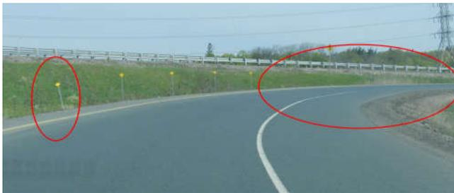
Figure 32 - Damaged Post-Mounted Delineators
