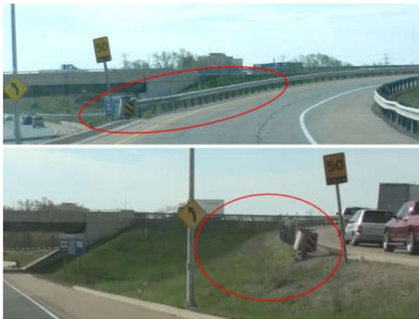
Figure 24 - Damaged and Poorly Designed Guide Rail End Treatment
