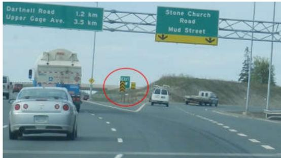
Figure 15 - Freeway Exit sign Partially Eclipsed by the Object Marker Warning Sign (View South from the Mainline)
