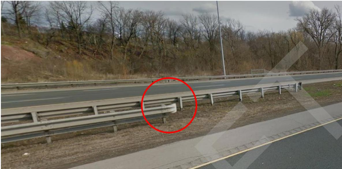
Figure 18: RHVP typical guide rail leaving end treatment
