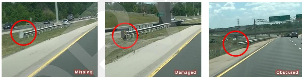
**Figure 24: Examples of Missing, Damaged and Obscured Object Marker Signs**
