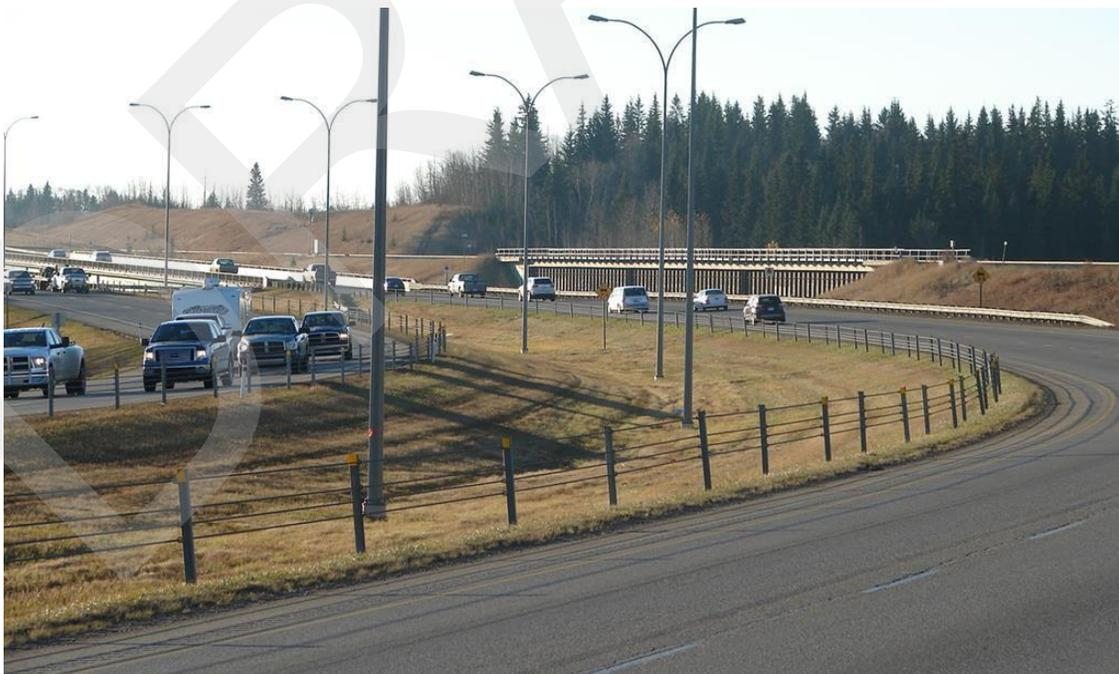
**Figure 31: Example of high tension cable barrier**
