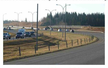
Figure 2: An Example High Tension Cable Barrier
