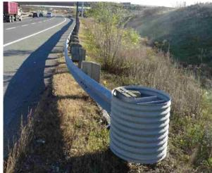
Figure 21: Substandard 4-inch Extruder
