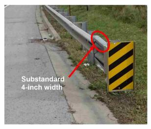
Figure 21: Substandard 4-inch Extruder
