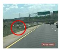
Figure 24: Examples of Missing, Damaged and Obscured Object Marker Signs
